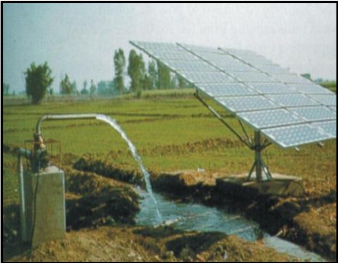
Fig: Solar Powered Tube well.
